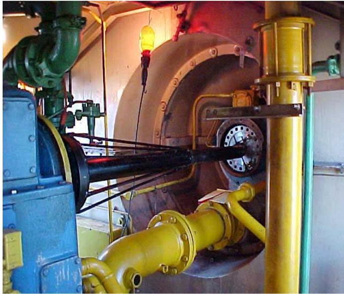
*The alignment fixture from gear box to the turbine*
